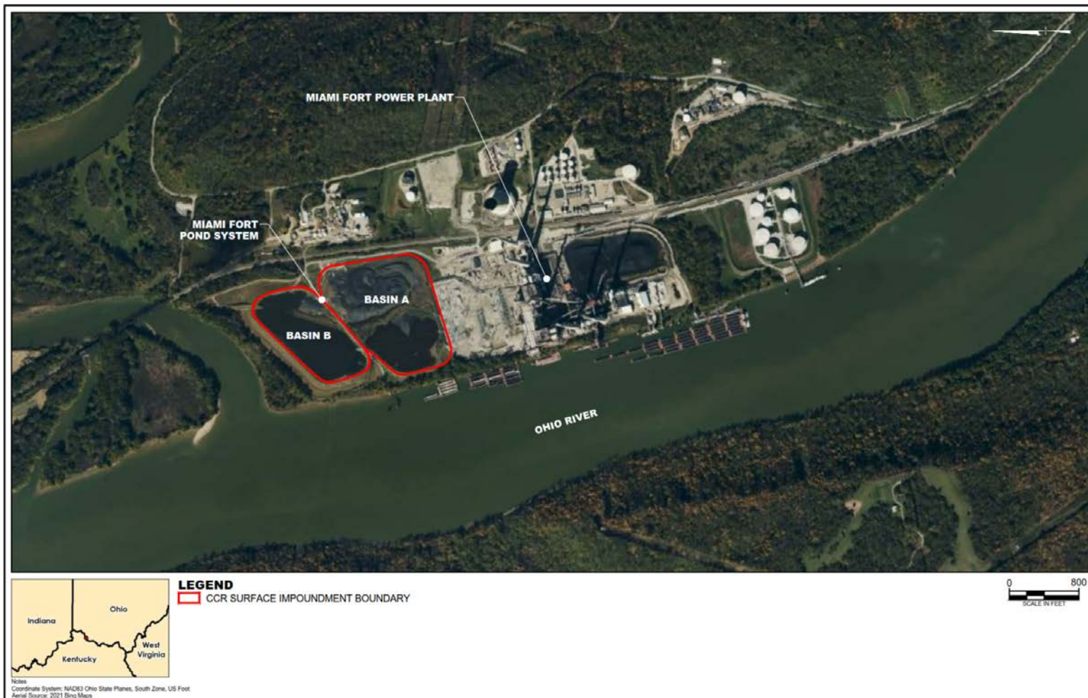
Figure 1-2. Miami Fort Power Plant CCR Impoundments & Related Facilities
